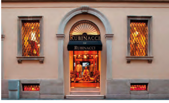
ATELIER RUBINACCI BUILDING - MILANO (ITALY)
