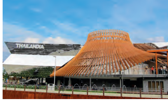
EXPO 2015 BUILDING - RHO Milano (ITALY)
