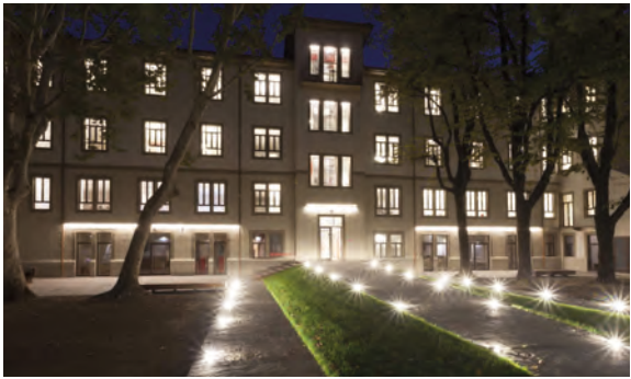
CASA EMERGENCY BUILDING - MILANO (ITALY)
